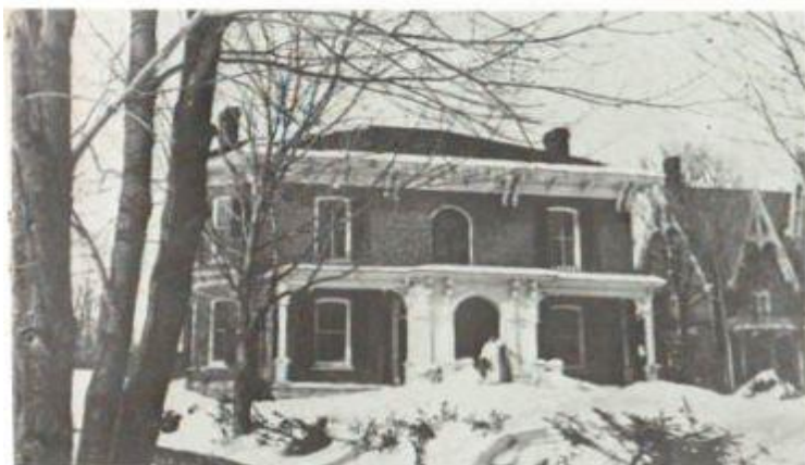
"Wexford": original verandah pictured here c. 1910, was much lighter in appearance than its replacement. This photograph also shows the original front sash, converted into French windows with fanlights in the c. 1917 alterations. (Courtesy Mr. and Mrs. Thomas Walker)
